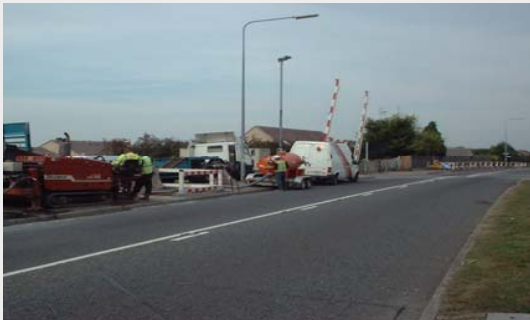
33kV Cable route rail track crossing
