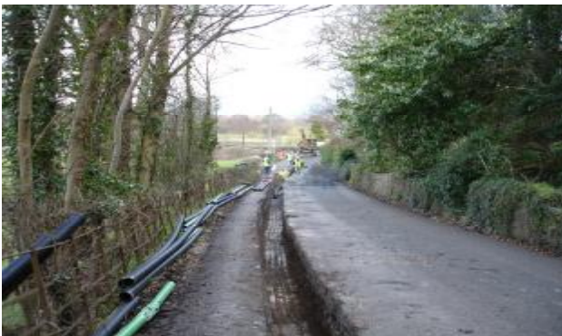
33KV GRID ROUTE UNDER CONSTRUCTION
