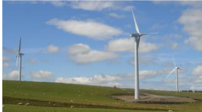
WIND TURBINES GENERATING WITHIN DAYS OF CONNECTION
