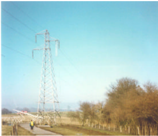
132kV Connection point
