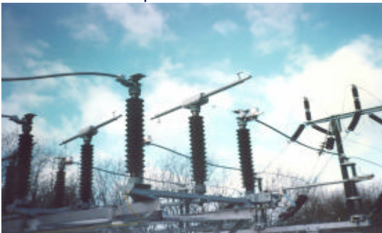
132kV Disconnectors
