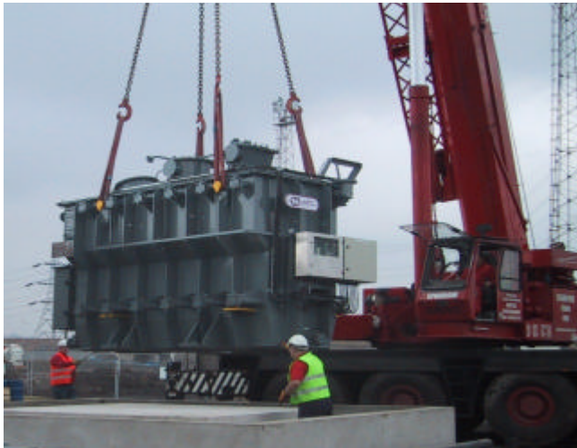
132/11kV 15MVA Transformer delivery
