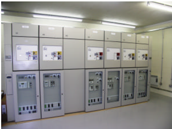
33kV switchboard
