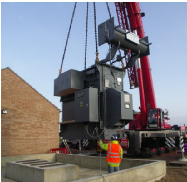
33/11kV 11/18/24MVA Transformer offload
