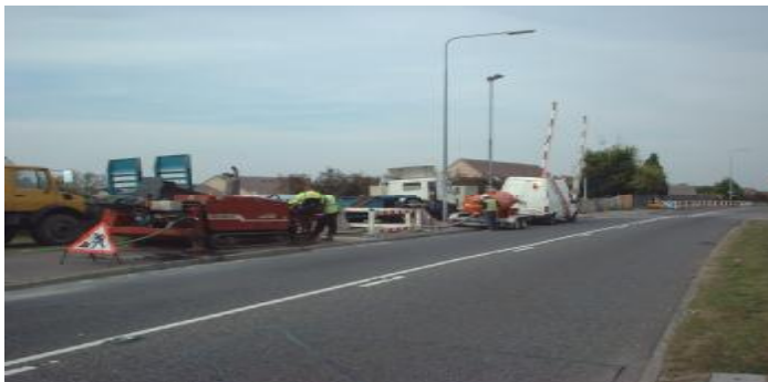
33KV CABLE ROUTE RAIL TRACK CROSSING
